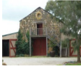
Barn/store to the north of the house.
