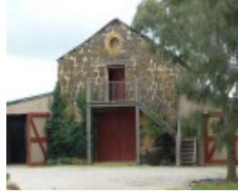
Barn/store to the north of the house.
