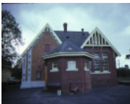
primary school number 461 burwood hwy burwood rounded wing sep1984
