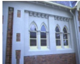
primary school number 461 burwood hwy burwood detail of windows
