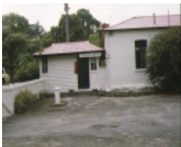
wattle park riversdale road surrey hills former stables and curator's office shelter
