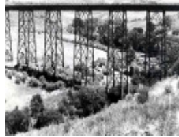
B5235 Railway Viaduct
