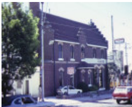
former es&a bank camberwell front view feb1982
