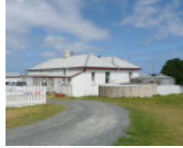
CAPE OTWAY LIGHTSTATION SOHE 2008
