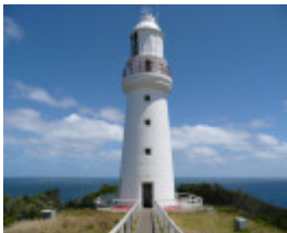
CAPE OTWAY LIGHTSTATION SOHE 2008
