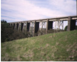
1 railway viaduct over moorabool river side elevation may1995
