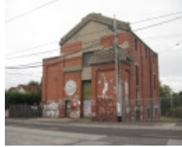
Ascot Vale Substation
