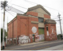
Ascot Vale Substation
