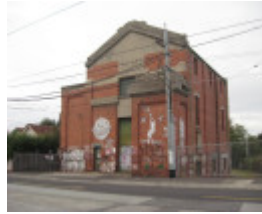
Ascot Vale Substation
