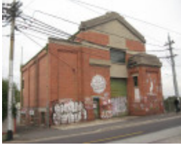
Ascot Vale Substation
