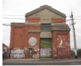
Ascot Vale Substation
