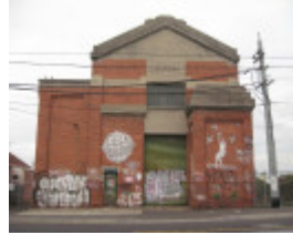
Ascot Vale Substation
