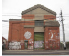
Ascot Vale Substation
