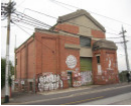
Ascot Vale Substation
