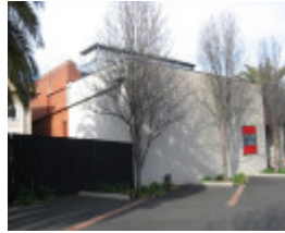
Elsternwick substation rear view
