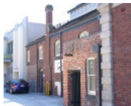
h01019 gordon technical college fenwick street geelong bldgd1 davidson hall she project 2004
