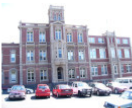
h01019 gordon technical college fenwick street geelong bldga administration bldg she project 2004
