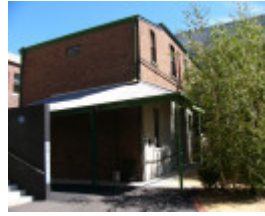
h01019 gordon technical college fenwick street geelong bldgf2 plumbing carpentry art modelling she project 2004
