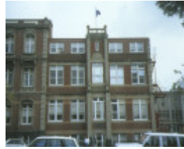
Gordon Technical College Geelong Front Elevation August 1995
