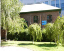
h01019 gordon technical college fenwick street geelong bldgf1 chemical laboratory she project 2004
