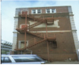
Gordon Technical College Geelong Exterior Staircase August 1995
