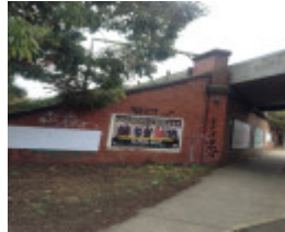
Rail over road bridge Ascot Vale Road
