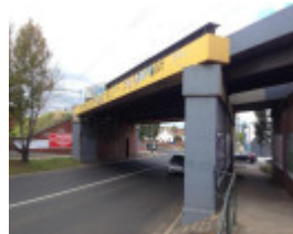
Rail over road bridge Ascot Vale Road
