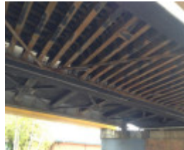
Rail over road bridge Ascot Vale Road
