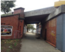
Rail over road bridge Ascot Vale Road
