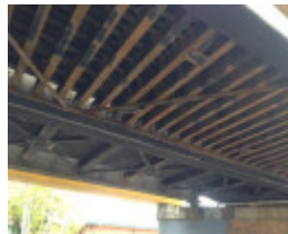
Rail over road bridge Ascot Vale Road
