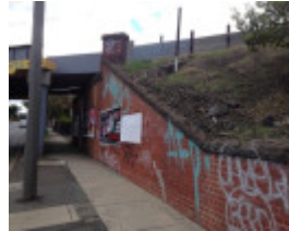
Rail over road bridge Ascot Vale Road
