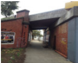
Rail over road bridge Ascot Vale Road
