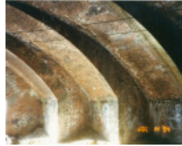
Dandenong Road Bridge. Source: National Trust of Australia (Victoria)
