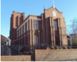
Tower Building, De La Salle College
