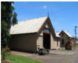
2013 stables coach house and dairy
