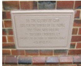
15-19 The Crossway, Strathmore
