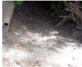
Brisbane St drain b
