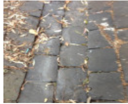
Bluestone drain Brisbane St and Ormond Rd
