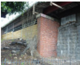
Racecourse Road Bluestone bridge abutment west side
