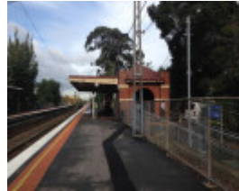
Newmarket Railway Station Down side building
