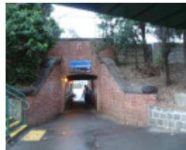
Newmarket Railway Station Pedestrian Subway east side
