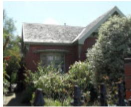
The Crescent 59 a
