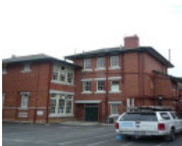
Essendon Primary School No.483 1922 block
