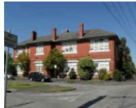
Essendon Primary School No.483 1922 school west elevation
