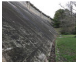
2017, dam wall (2).jpg
