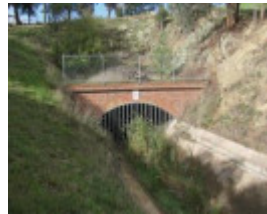
2011, brickwork to tunnel 4.gif
