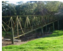
2011, Plenty River pipe bridge.gif
