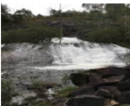
2017, base of spillway.jpg
