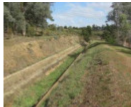
2011, decommissioned aqueduct, central section.gif
