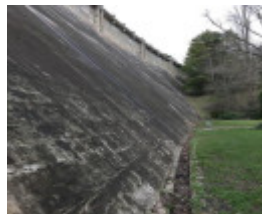
2017, dam wall (2).jpg
