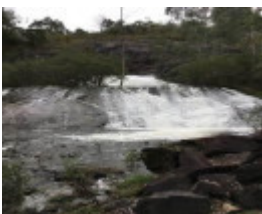
2017, base of spillway.jpg
