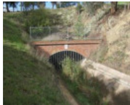
2011, brickwork to tunnel 4.gif
