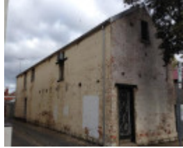
House, dairy and stables 41 Moore Street
