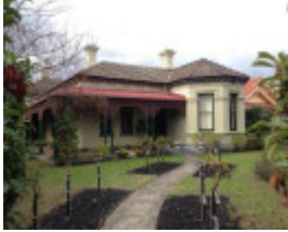
House, dairy and stables 41 Moore Street
