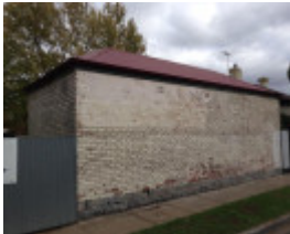
House, dairy and stables 41 Moore Street
