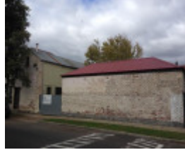
House, dairy and stables 41 Moore Street
