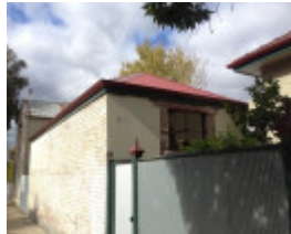
House, dairy and stables 41 Moore Street
