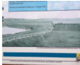
Holmes Road drain outlet 1920 Historic photograph
