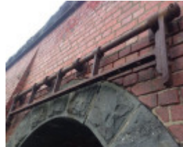
Holmes Road drain outlet
