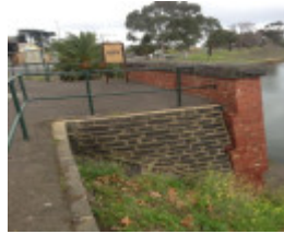
Holmes Road drain outlet
