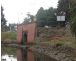
Holmes Road drain outlet
