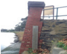
Holmes Road drain outlet
