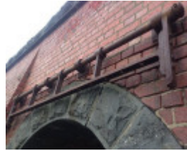
Holmes Road drain outlet
