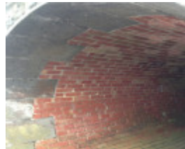
Holmes Road drain outlet
