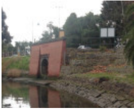
Holmes Road drain outlet
