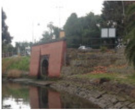
Holmes Road drain outlet
