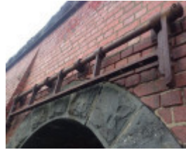
Holmes Road drain outlet
