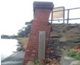
Holmes Road drain outlet
