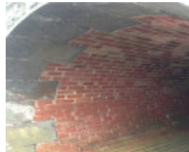
Holmes Road drain outlet
