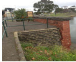
Holmes Road drain outlet
