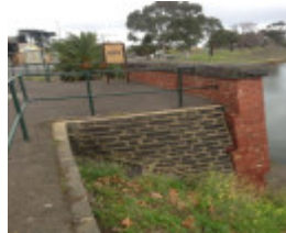
Holmes Road drain outlet
