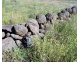
Dry Stone Wall B118
