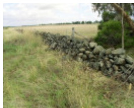
Dry Stone Wall B123
