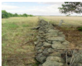
Dry Stone Wall B123
