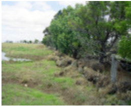
Dry Stone Wall B125
