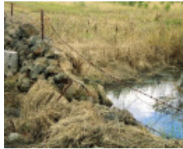
Dry Stone Wall B126
