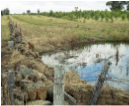
Dry Stone Wall B126
