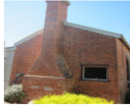
131 Goynes Road, kitchen & chimney at rear of house
