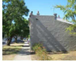
105 Lucan Street, side view
