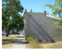
105 Lucan Street, side view
