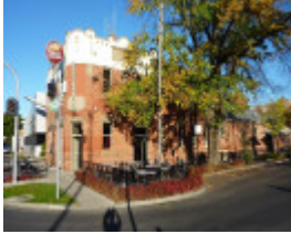
View of the north elevation, extending along Water Street
