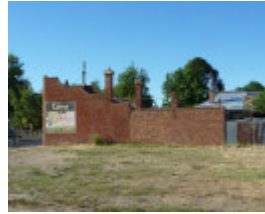
Property as viewed from the north
