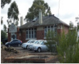
The main building of the former Bendigo East school, viewed from the east
