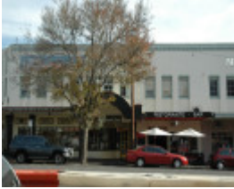
58 Moorabool Street, Geelong
