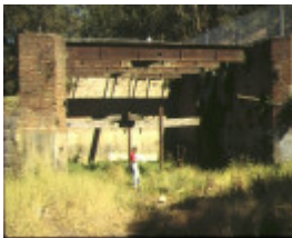
dights mill site dights falls abbotsford front view of mill dec1994
