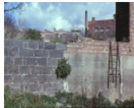
dights mill site dights falls abbotsford wall detail aug1979
