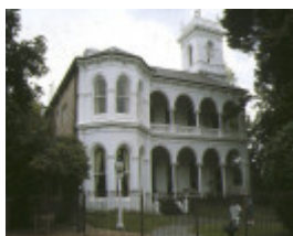
1 cullymont selwyn street canterbury front view
