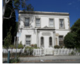
52 Albion Street, South Yarra
