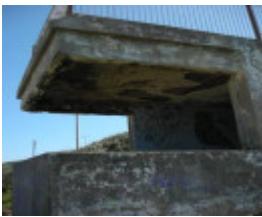
2018, World War II bunker on southern boundary.jpg
