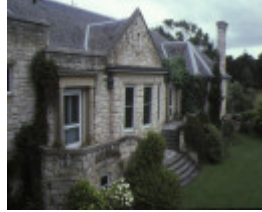
barragunda cape schanck road cape schanck new wing dec1984
