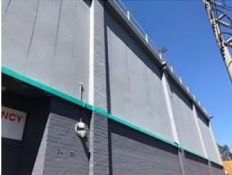
2018, details showing concrete panels.jpg
