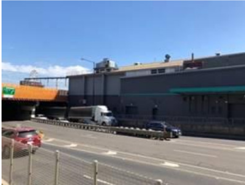
2018, Dudley Street from south-east.jpg
