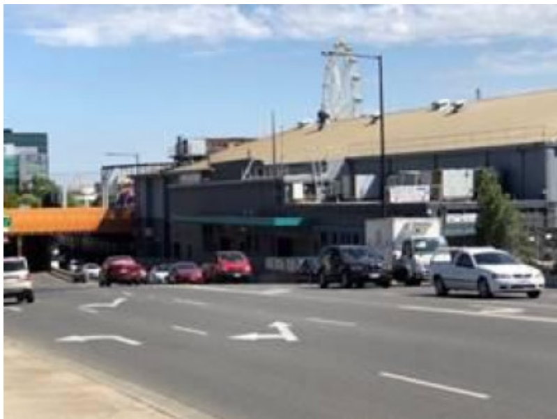
2018, Dudley Street from south-east 2.jpg
