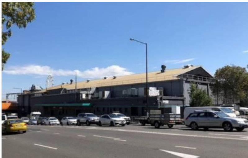
2018, Dudley Street elevation.jpg
