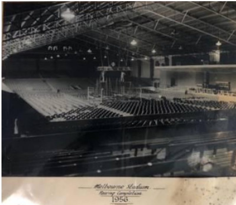
1956, interior nearing completion.jpg
