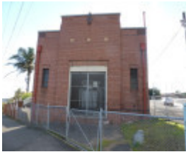
Brunswick West Tramway Substation
