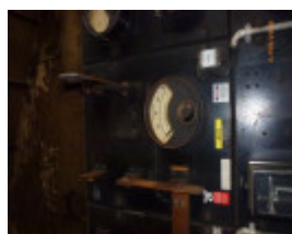
Switchboard meter
