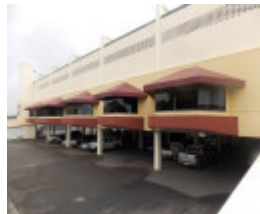
General view of the 1976 additions from west (carpark side), looking north-east.jpg
