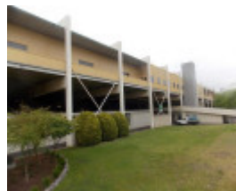
General view of the grandstand from west (carpark side), looking south-east.jpg
