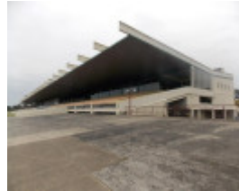
from east (trackside), looking south-west.jpg
