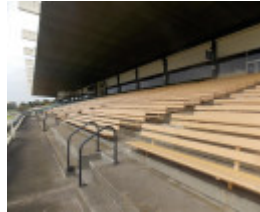
Detail of seating area, showing stepped concrete tier, bench seats and canopy underside.jpg
