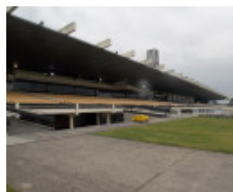
view of the grandstand from east (trackside), looking north-west.jpg
