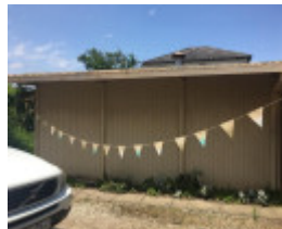
Grant House 2018, West facing elevation (rear module).jpg
