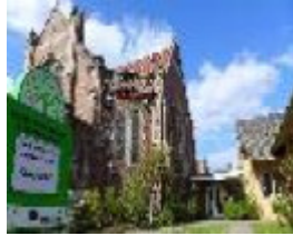
St David's Uniting Church, 902A Burke Road east
