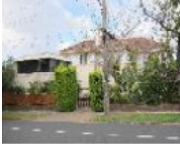
486 Burke Road, seen from Pine Avenue.
