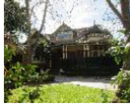
View Street 15 (2).jpg
