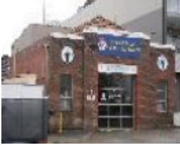
Canterbury Road, 61 CANTERBURY AMBULANCE STATION
