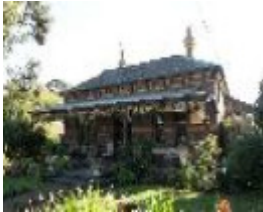
35 Chatham Road, Canterbury KAIAPOI
