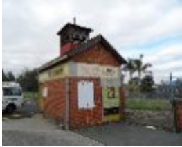
Substation at 6 Harp Road, Kew.
