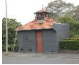
Substation at 190A Canterbury Road, Canterbury.
