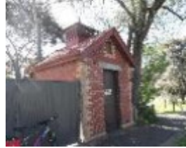
Substation at 26A Myrtle Road (next to 37 Canterbury Road), Canterbury.
