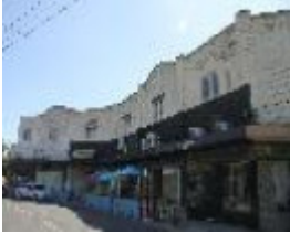
Fordham Avenue, 112-128 Hartwell Hill Shops
