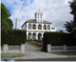
Aberfeldie Street and Waverley Street Precinct
