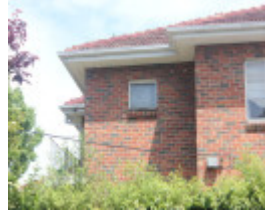
62 Napier Crescent Essendon
